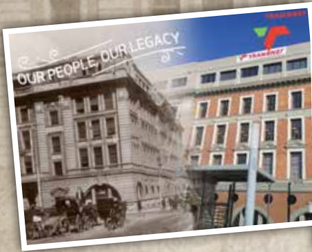
Transnet's Head Office Building 96 Rissik Street Head Office - JHB. Built: Early 1900s
